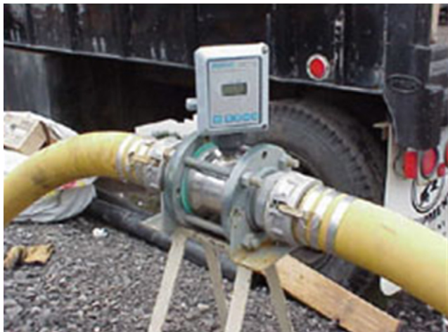
Fig. 5. Grout-flow meter in operation.
