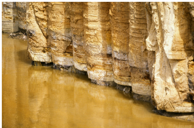
Fig. 8. Exposed stabilised soil-cement wall.
