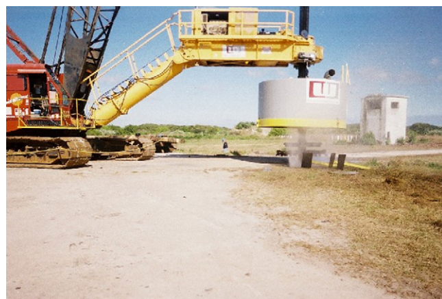
Fig. 7. Drill rig equipped with a hood.
