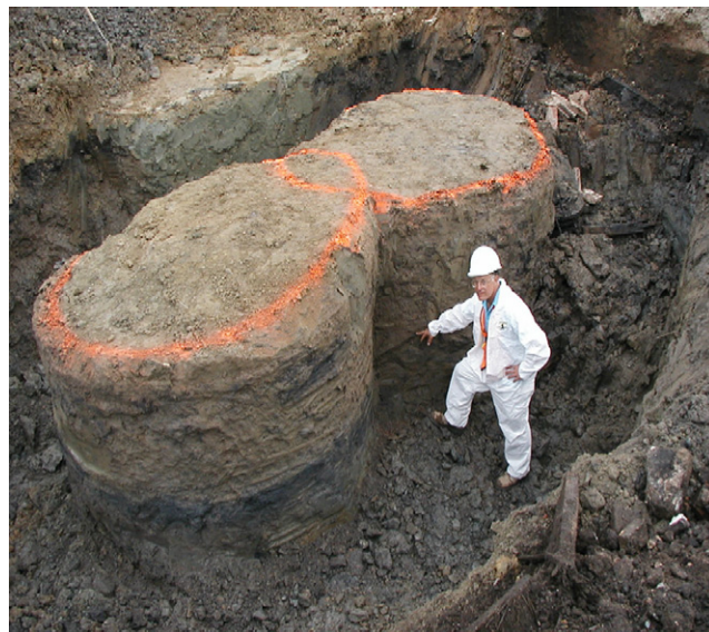
Fig. 4. Example of mixed column geometry.
